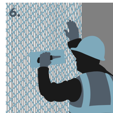
Applying reinforcing mesh.
