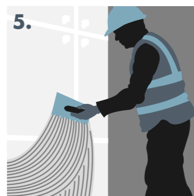
Applying notches within basecoat.
